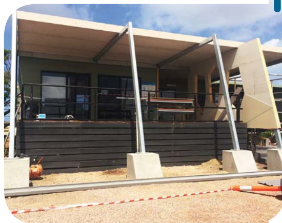
Building the roof over the deck
