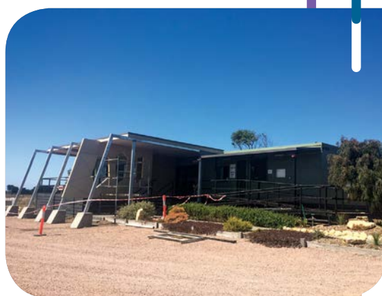
Side view of the construction
